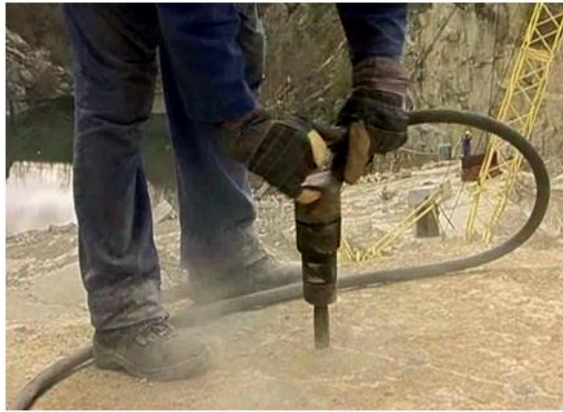
FIG. 5 - EXAMPLE OF OPERATION WITH HAND-TRANSMITTED VIBRATION TO THE UPPER EXTREMITIES – STONE QUARRY
